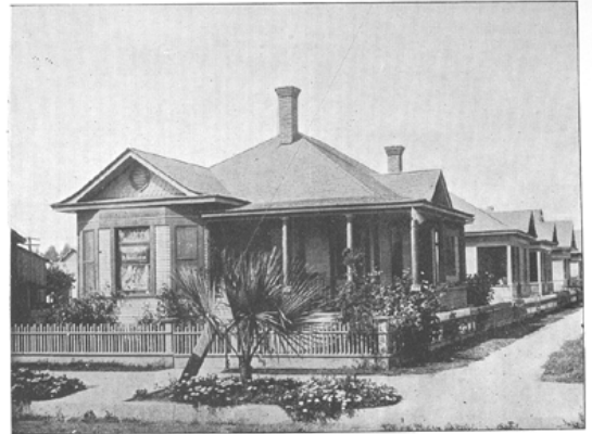
From the early 1900s; a house at 5 th & Pine.
