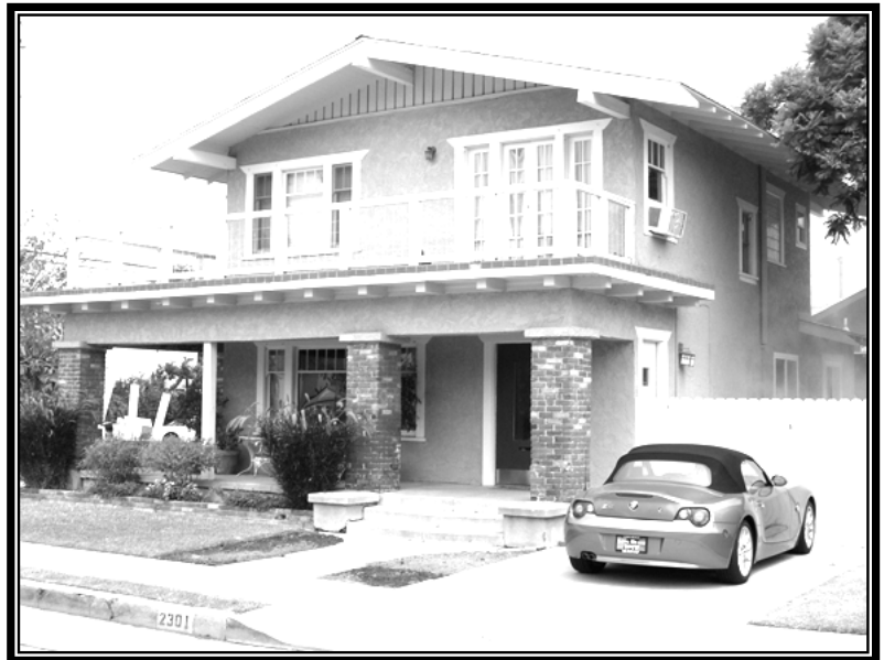
Before stucco removal.
