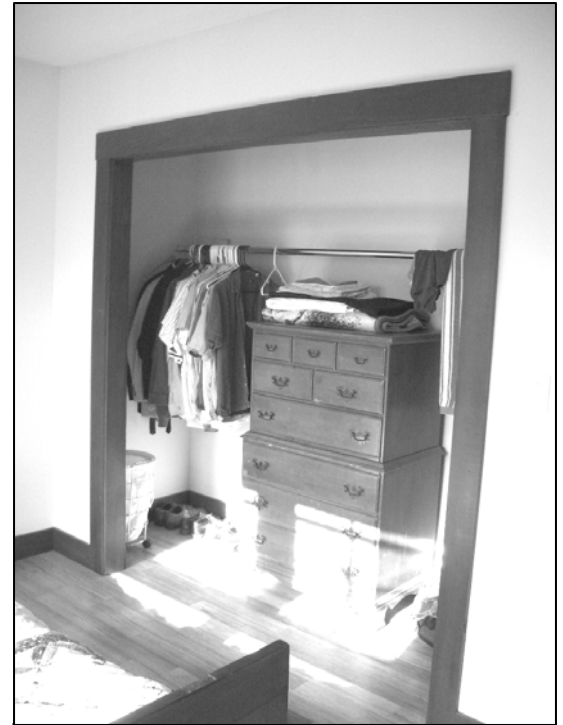
Historic-look trim is added to a remodeled closet so it fits the “look” of the house.
