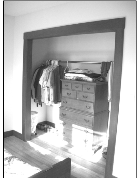
Historic-look trim is added to a remodeled closet so it fits the “look” of the house.
